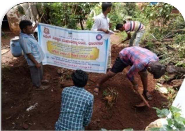
Construction of toilet taking place in Yerikoppa Grama.
